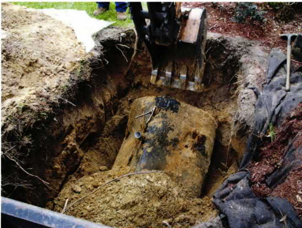
Picture 2: UST 1297Eagle removal in progress.
